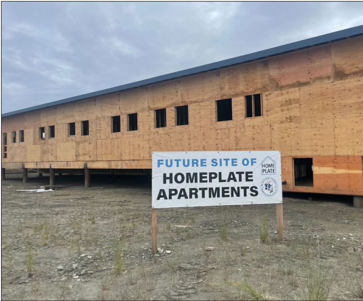
The Homeplate Nome Apartments construction site. Photo by Ava White.
